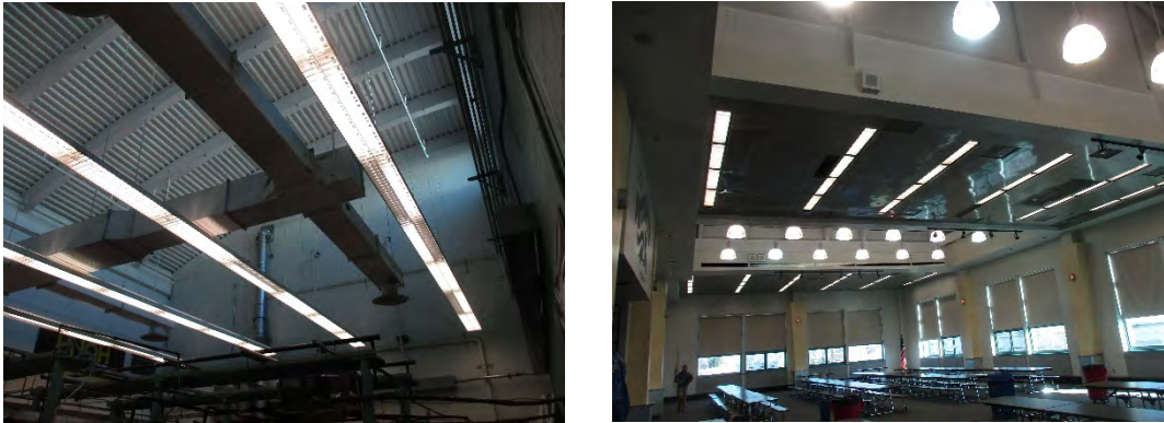
Examples of existing interior lighting
