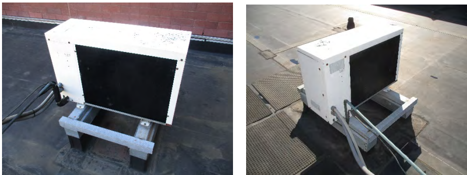
2D.1 Existing Split System Units to be Replaced
